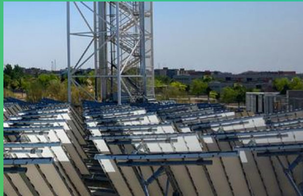
CEMEX – Solar Clinker
